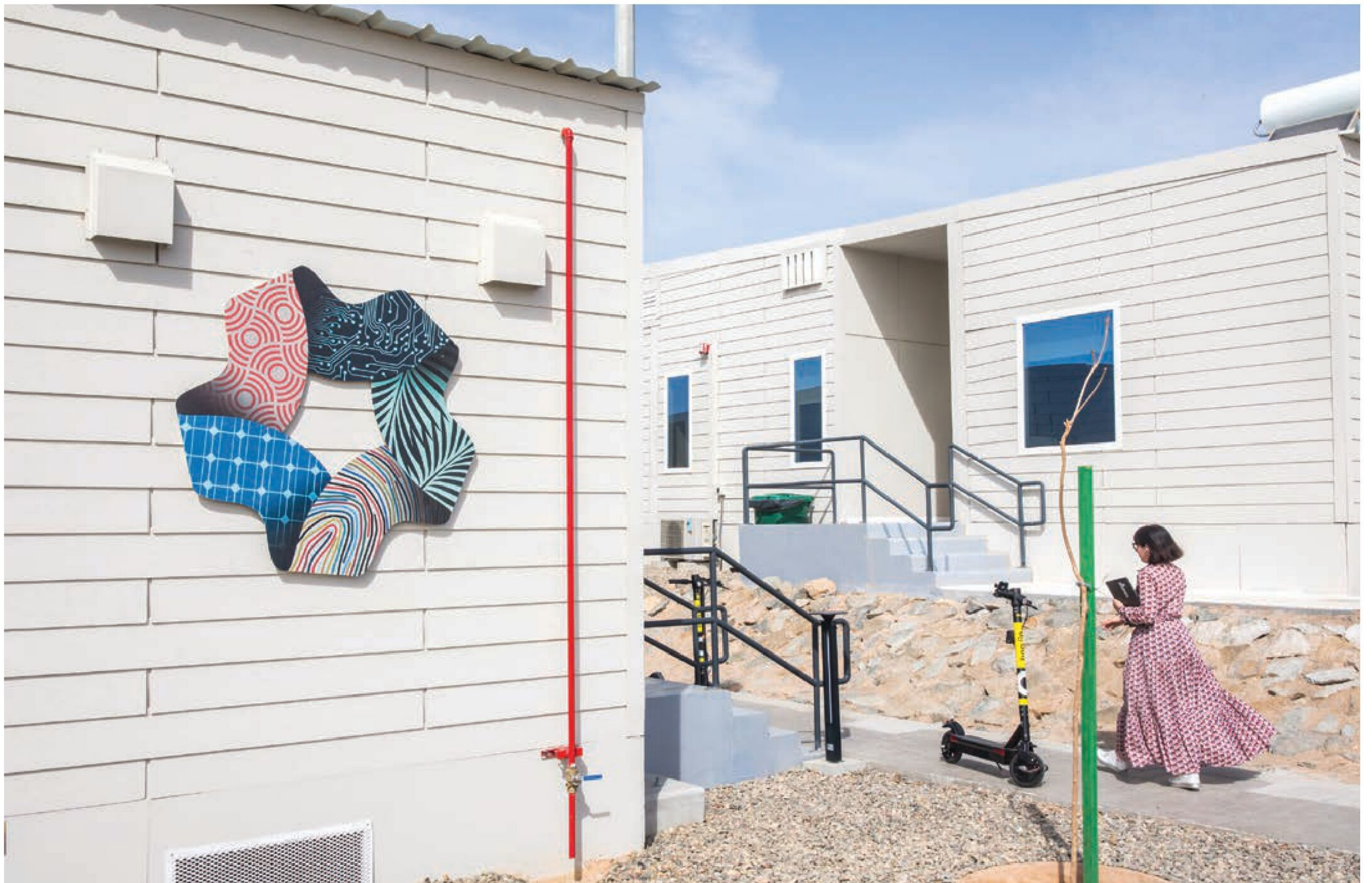
▲ Temporary office buildings
